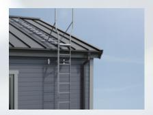
Durable steel ladders for fixed mounting on walls and roofs. It is suitable as a roof ladder at all heights and as a wall ladder on properties where the facade is a maximum of 8 meters. It can also be used on chimneys and similar constructions without any height restrictions.
